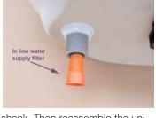
replace it in the fill valve shank. Then reassemble the universal waher, friction washer, and coupling
